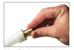
Insert fitting into expanded tube and sleeve. Hold fitting in place until tube/sleeve constricts annularly around the fitting.
